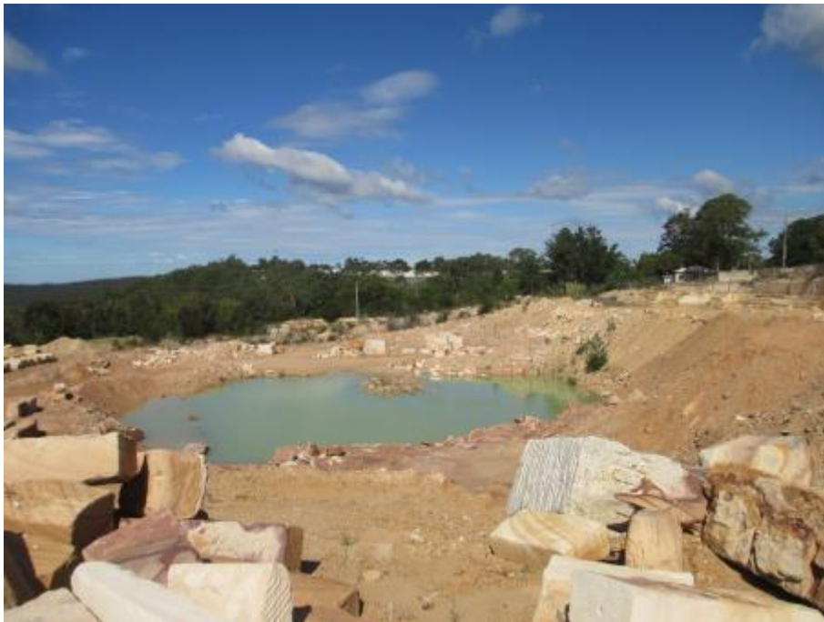
Photograph 6: Small on Site settling pond located in the western portion of the Site. Photograph taken looking south.
