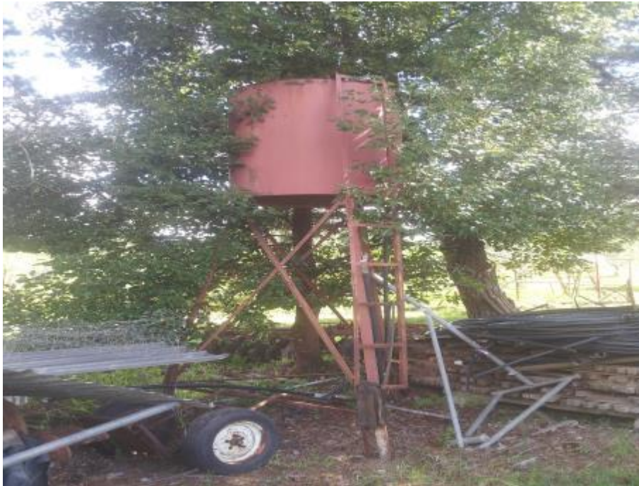
Photograph 22: Above ground storage tank (AST) observed in the central portion of the Site. The contents and volume of the AST was unknown.
