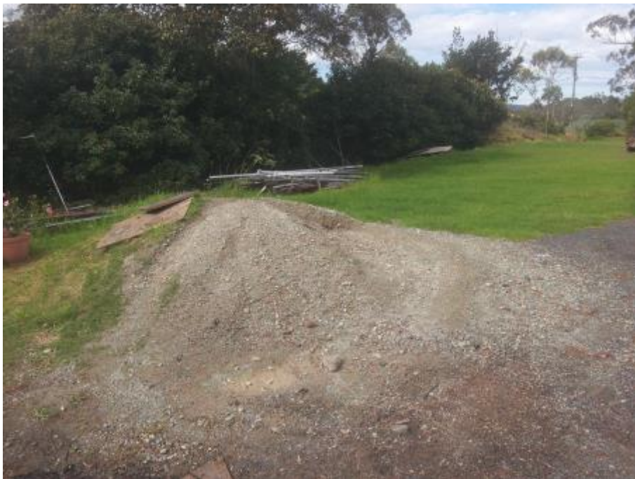
Photograph 28: Fill mound located to the east of the workshop/storage shed. The fill mound was noted to contain gravelly clay material assumed to be used for the construction of the Site driveway. Photograph taken looking north east.
