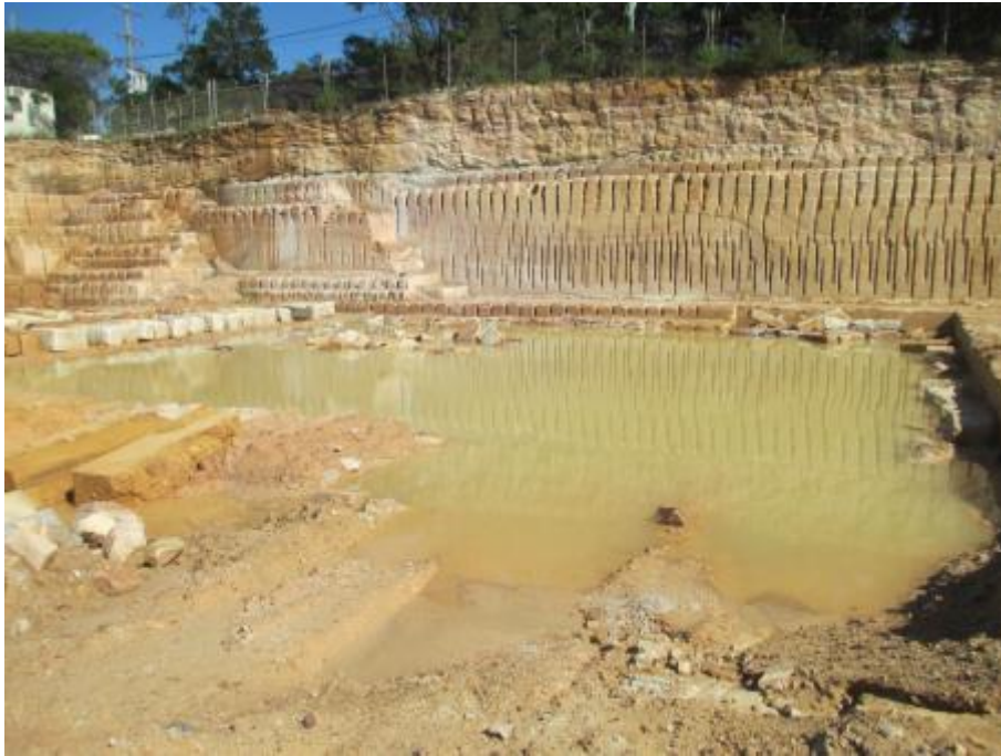
Photograph 5: Example of surface water pooling observed on Site. Photograph taken looking west.
