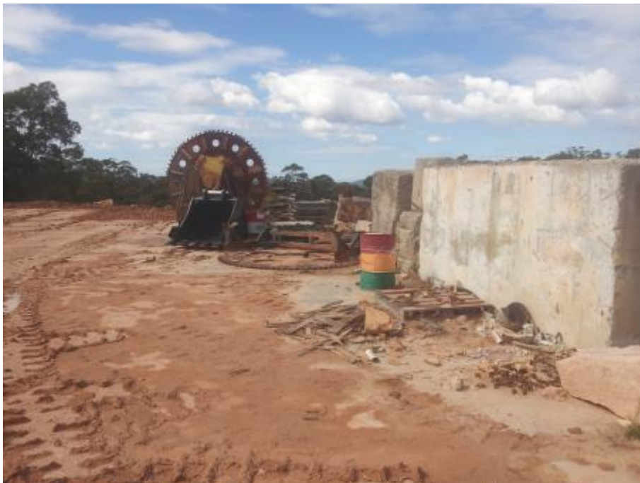
Photograph 14: Concrete pad located in the north eastern portion of the Site. According to the quarry manager, this area is currently used for the storage or quarrying equipment in addition to the maintenance and re-fuelling of machinery.
