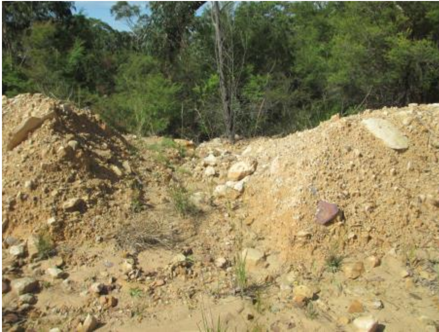
Photograph 11: Example of surface water runoff occurring through gaps in bund wall bordering the southern margin of the main quarry area. Photograph taken looking south.
