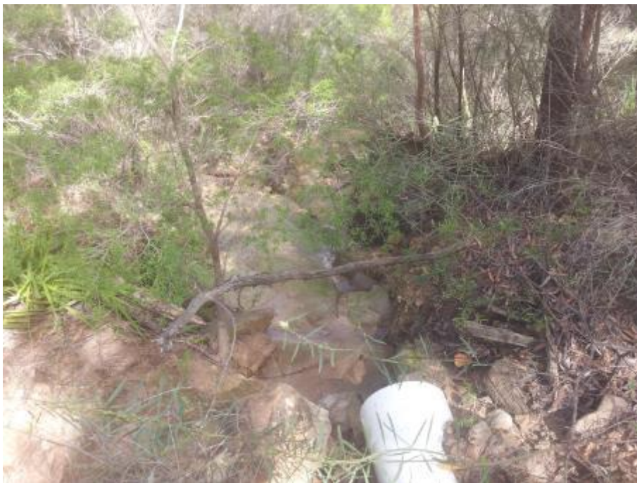
Photograph 10: Large diameter drainage pipe directing surface water seepage from large on Site settling pond to back-up settling ponds located to the south of the main quarry area.
