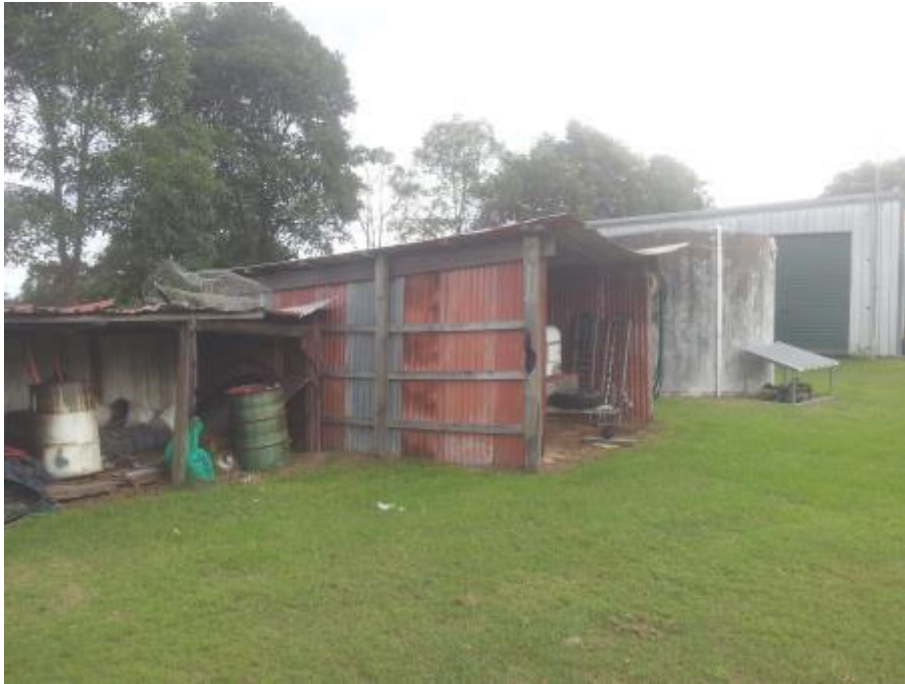
Photograph 32: Small storage sheds located to the south of the large white storage shed. These sheds were noted to contain assorted stored materials and assorted farm equipment.
