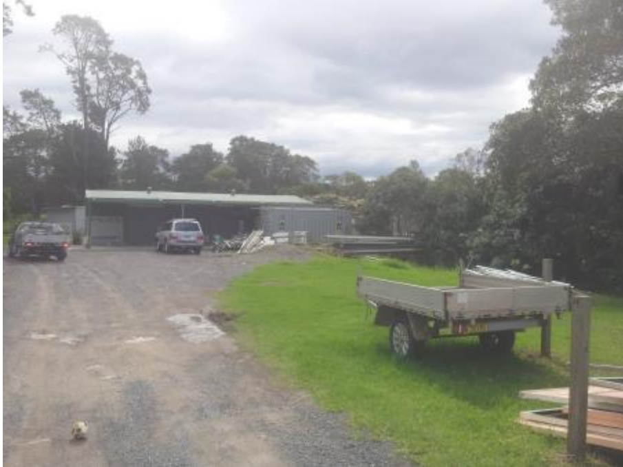
Photograph 25: Workshop/storage shed located in the eastern portion of the Site. Photograph taken looking north west.
